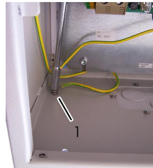
Figure 5-19: Removal of Ground Wire
